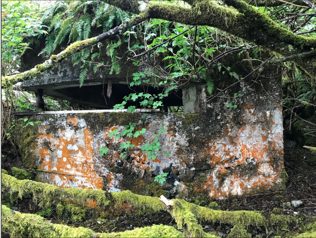
Photograph 1: Northwest Exterior of Observation Post (May 2020)
