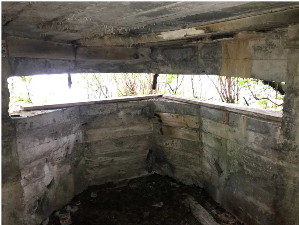
Photograph 2: Interior of Observation Post (May 2020)
